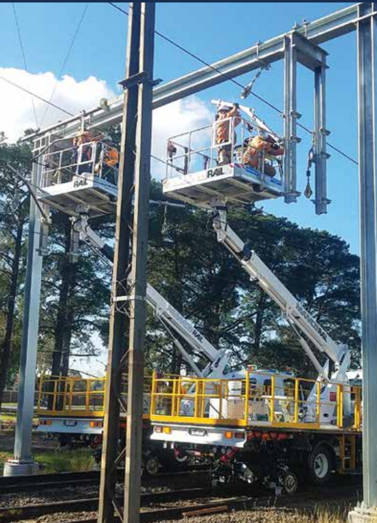
Manco EWP Rail Trucks working on the Melbourne contract
